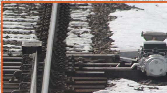
Nearly **5,000** switch heaters are in place to ensure remote-controlled rail switches do not freeze.
