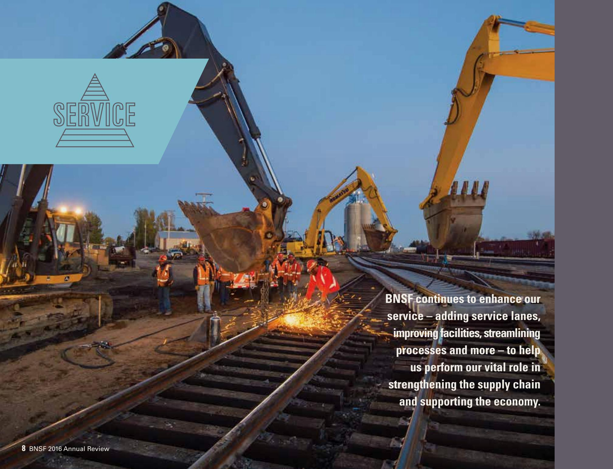
A large-scale construction site for a railroad at dusk. Several yellow excavators are positioned around the tracks. In the foreground, a worker in a red jacket is welding a rail joint, creating a bright orange glow. Other workers in orange safety vests are visible in the background. The sky is a deep blue, and the scene is illuminated by the warm light of the setting sun and the bright sparks from the welding process.
